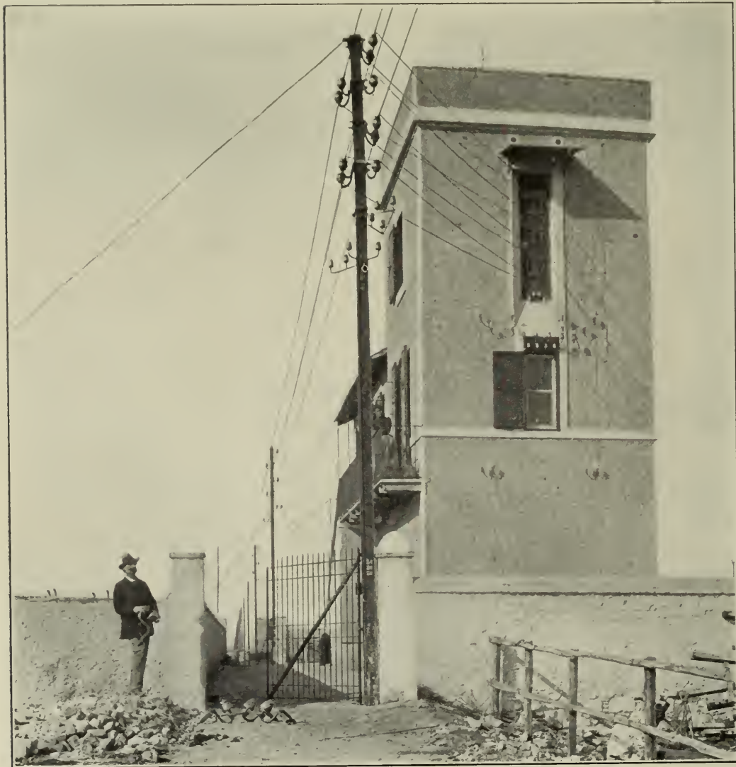
FIG. II. THE "CAPANNACCE"—MEASURING AND LINE-PATROL STATION ON THE LINE FROM TIVOLI TO ROME.
